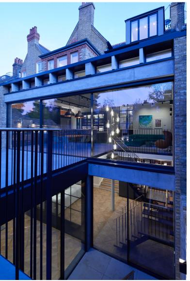
The L2i-S650 Slimline Sliding Doors are the ideal solution for projects requiring wide spans with minimal aluminium sight lines. They are capable of weights of up to 600kg on the manual sysytem and on the automated system up to 700kg.
